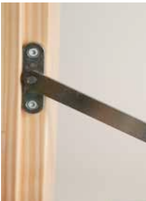
Handle operated hold open friction stay for SHID.
