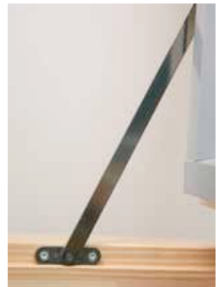
Handle operated hold open friction stay for SHI.
