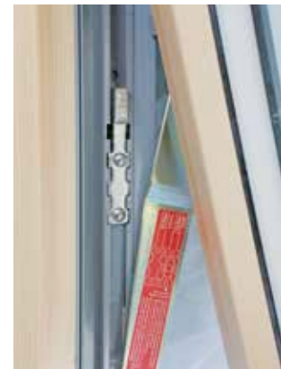
For TSG180 Integral restrictor.
