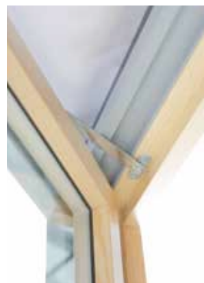
Handle operated friction stay (hold open device) for SHG model only.
